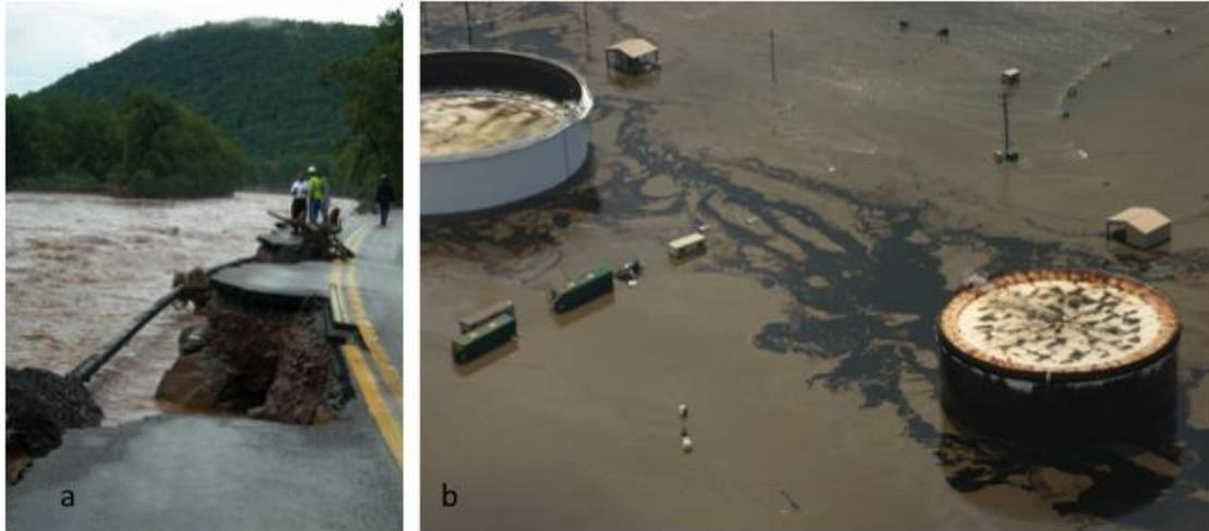
**Fig 3: a) Damage to pipe due to flooding of Pennsylvania, USA, 2004 [source: <https://dcbureau.org/tag/earthjustice>]; b) hydrocarbon release in an oil refinery after the flooding of Coffeyville (USA), 2007 [source: <http://ksview.org/info/news.shtml>].**
