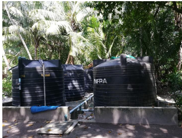
Figure 2. Public water tank used by the inhabitants of Magoodhoo to collect rainfall water for daily use.
