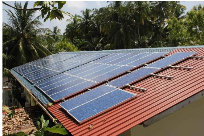
Figure 6. Photovoltaic plant under construction on the rooftop of Magodhoo Municipality.
