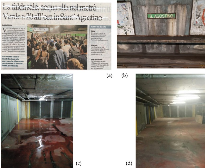
Fig. 5.12. a) Newspaper article of “La Repubblica” (2 nd July 2013), dealing with flooding episodes in Sant’Agostino station. b) Flooding evidence in Sant’Agostino station (8 th September 2020). (Image credits to the authors). c) Flooding evidence in Numa Pompilio public car park. d) Absence of flooding evidence after waterproofing works in Numa Pompilio public car park. c) and d) : images were provided by Rete Irene.
