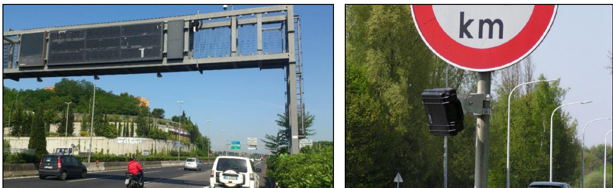
Figure 4. A variable Message Panel (left) and a traffic counter on a road sign (right).
