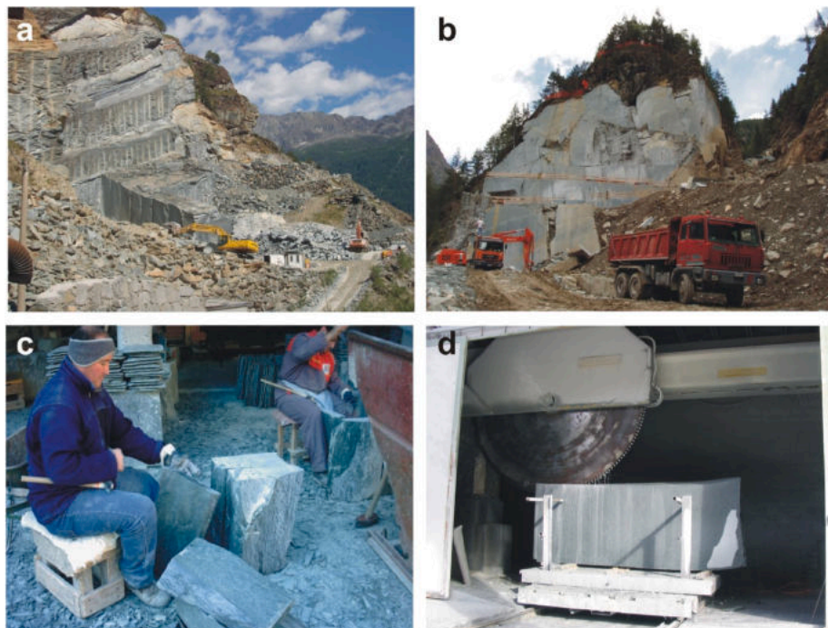
Fig. 3. a) Sasso Corvi schistose serpentinite quarry; b) Valbrutta “massive” serpentinite quarry; c) traditional manual splitting by hammer and chisel in thin slabs; d) Diamond disc cutting of a “massive” serpentinite block.
