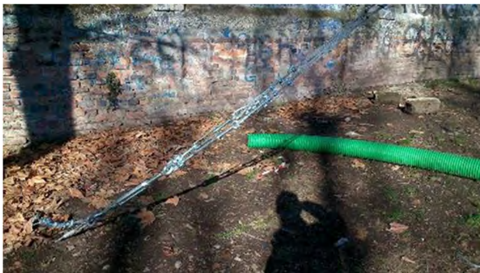
Fig. 7.15 Phase 6 - Final system of tensioners
