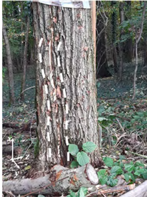
Fig. 5.16 Crack formation during the Test 2.
