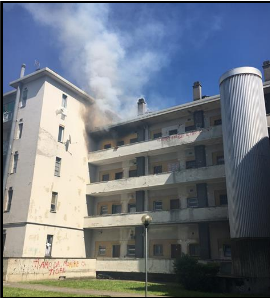
FIGURE 5-11 - FIRE AT VIA ABBIATI, 6
