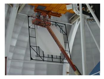
**Figure 8.4:** Installing the existing reflection screen used for daytime flat fielding. The screen is being mounted to the inside of the dome, between the arch girders and just below the attachment point for the dome crane rails. Note the use of a long-reach boomlift. For safety reasons, the telescope drives must be locked out and tagged out during the entire operation.
