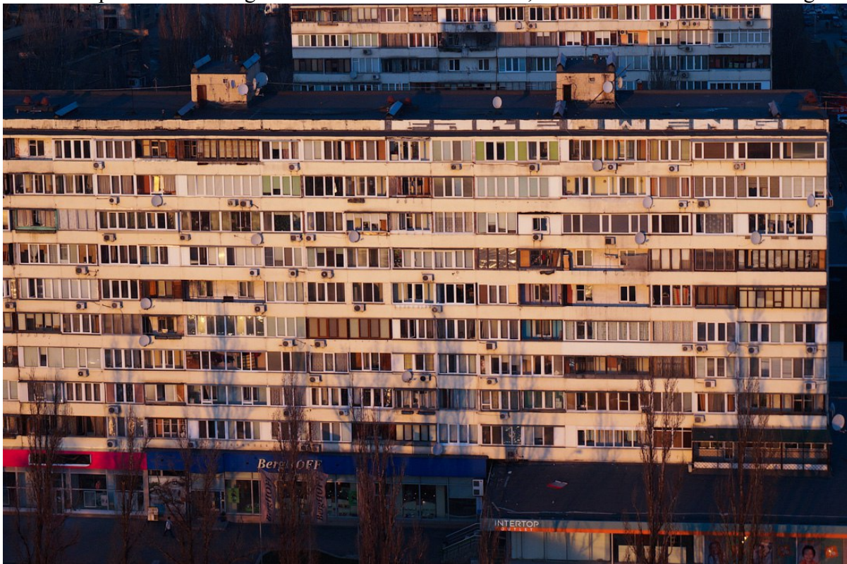
Photo 1. Apartment housing with self-renovated balconies, insulation and air conditioning
