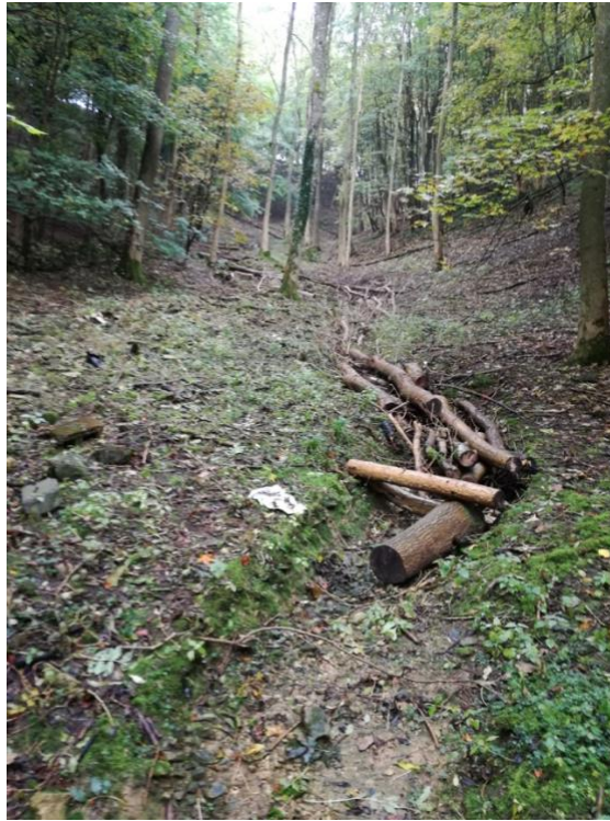
Figure 6. 12 Gulley stuffing in the Painswick valley
