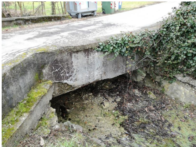
Figure 6. 18 LOII reported that this bridge over the Bertolini stream was 1.5m high in the past
