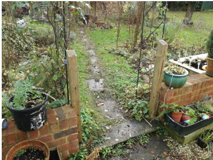
Figure 6. 6 Individual property protection (wall and bulkhead) built by the EA in front of FG4 house
