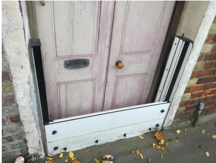
Figure 6. 5 Individual property protection (bulkhead) built by the EA at the bottom of the Slad Valley
