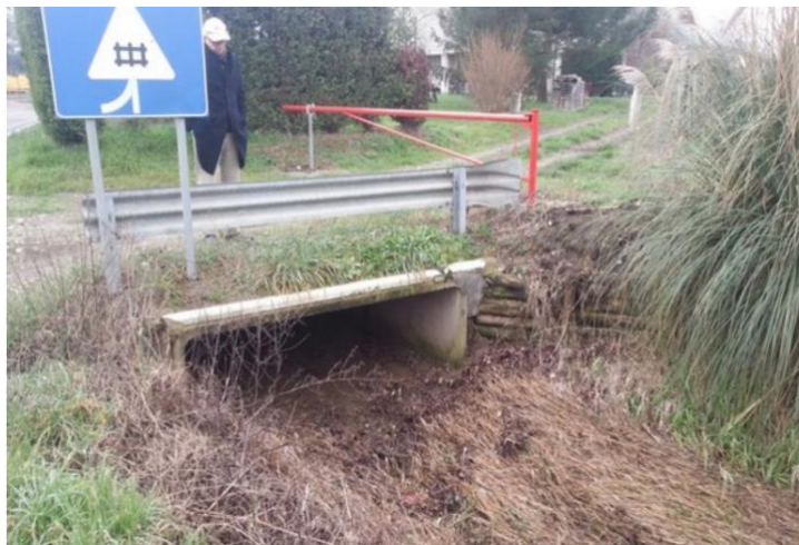
Figure 6. 22 The Rio Montefalcone channeled and culverted in the middle of Bibbiano town (source LIFE RII)
