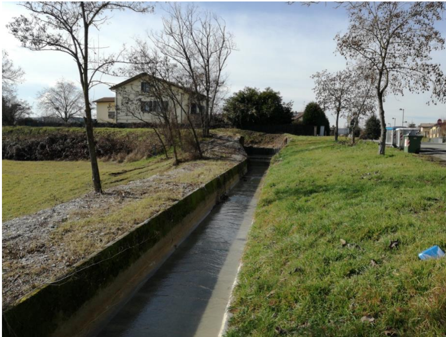
Figure 5. 8 The Rio Enzola flows like a channel and is elevated above the ground level (on the left side)
