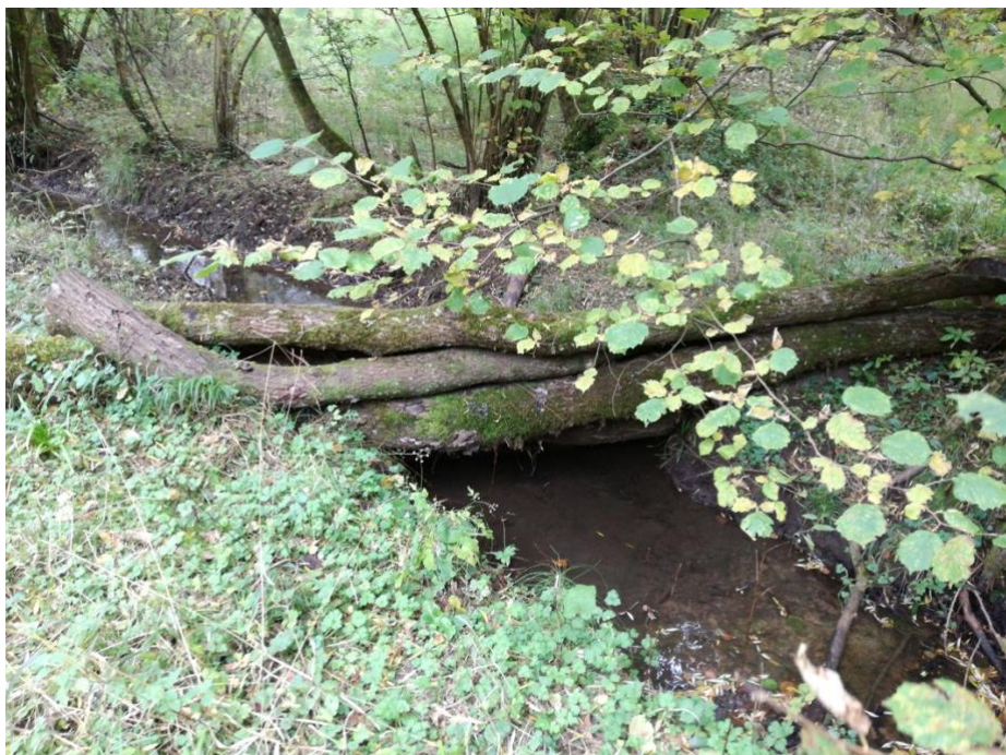
Figure 6. 8 Leaky dams built with tree trunks in the Slad brook
