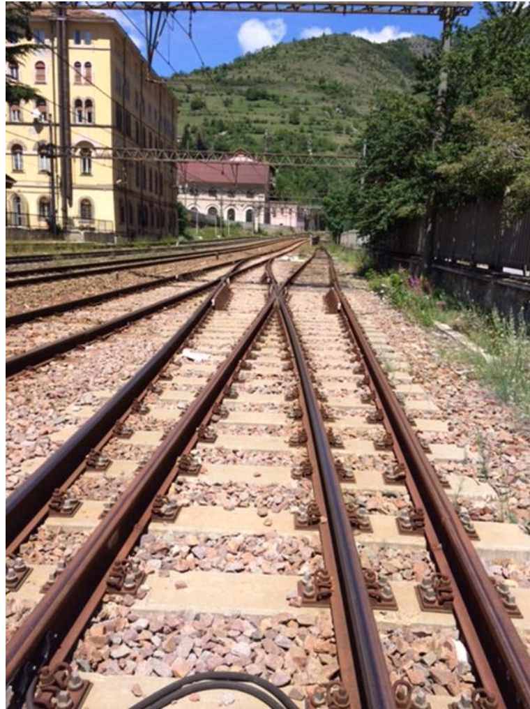
Figure 29: Example of a railroad switch 58
