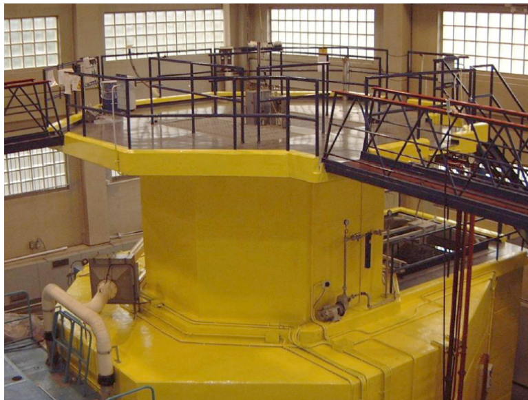
Fig. 2.1: The TRIGA Mark II reactor at the Applied Nuclear Energy Laboratory of the University of Pavia.
