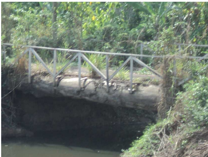
The bridge built by Togo
