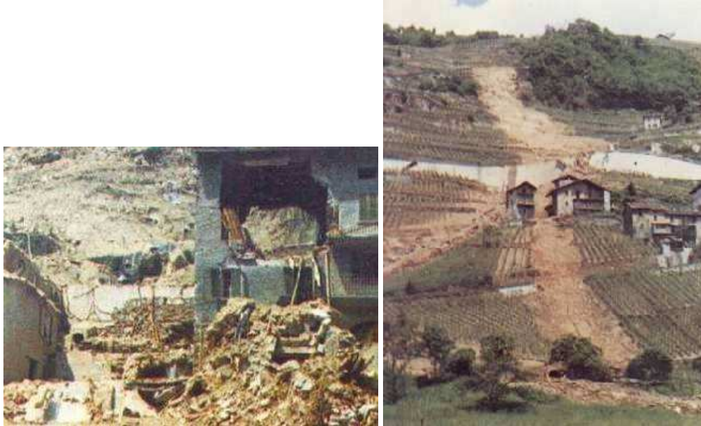
Figure 2.5. Consequences of the landslides of May 1983, a) buildings destroyed by the debris flow in Tresenda; b) debris flow in Valgella.
