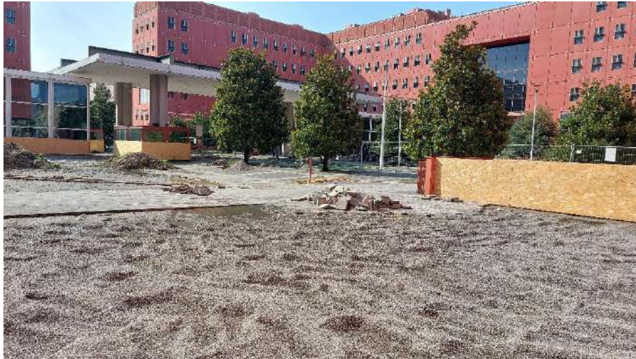
Figure 3.15. Overview of part of the square during the depaving work.
