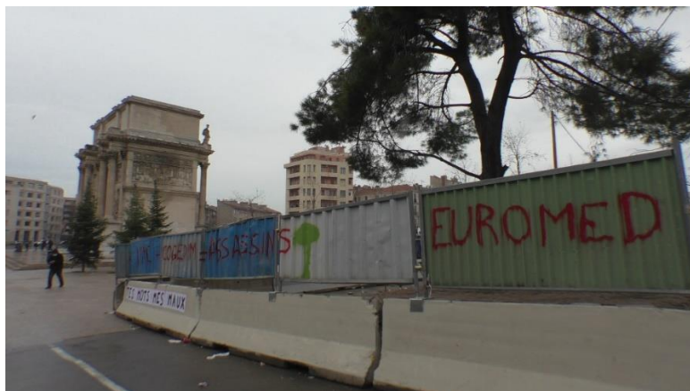
Figure 21. Euroméditerranée urban renewal project in the centre of Marseille
