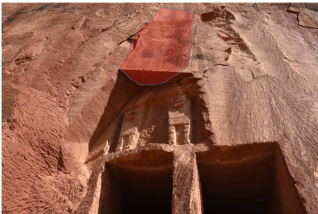
Fig. 20 Potential collapse in the quarried part of the slope and involving archaeological remains
