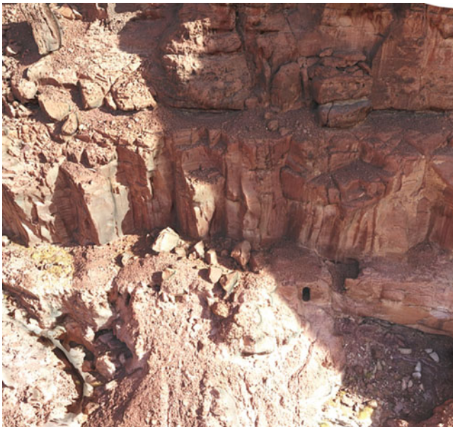
Fig. 16 Example of rockfall affecting the rocky cliff of Dadan
