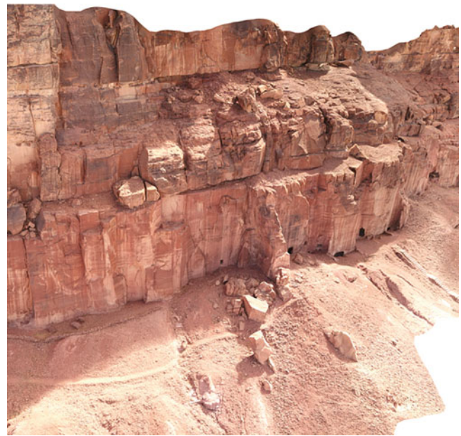
Fig. 21 Collapsed blocks at the toe of the cliff with the pedestrian pathway passing through. This is a clear example of a pathway standing too close to the cliff and exposing visitors to a potential risk of being involved in a rockfall
