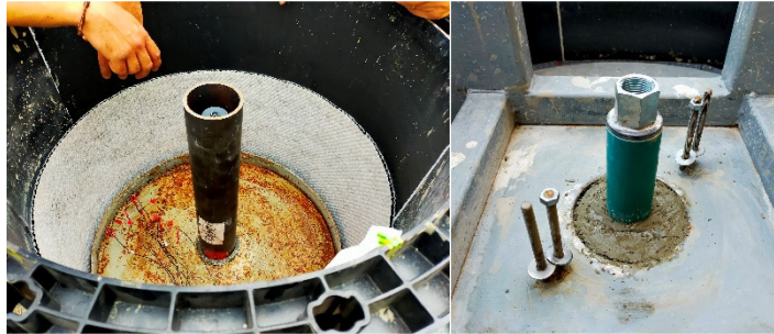
Figure 21: cylindrical machine, on the left it's possible to see the casing for bentonite sheath, on the right the top of machine.
