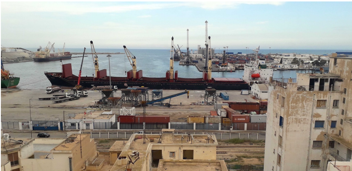
Fig. 1 View of Sfax port from top floor of Hotel Les Olivier Palace (photograph by Dines, 02/06/2023)
