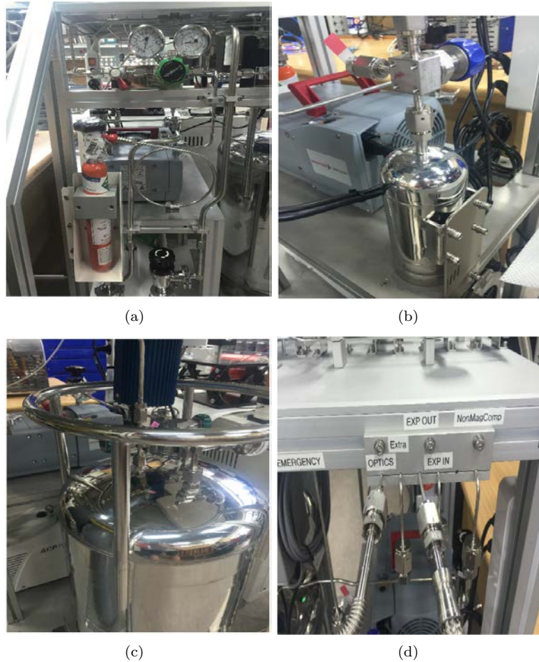
Figure 5: Part of gas handling system
