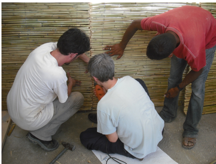
Source(s): Figure reproduced with permission from ©ARCò
