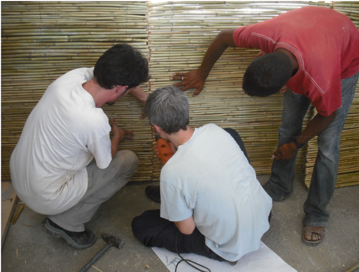
Source(s): Figure reproduced with permission from ©ARCò
