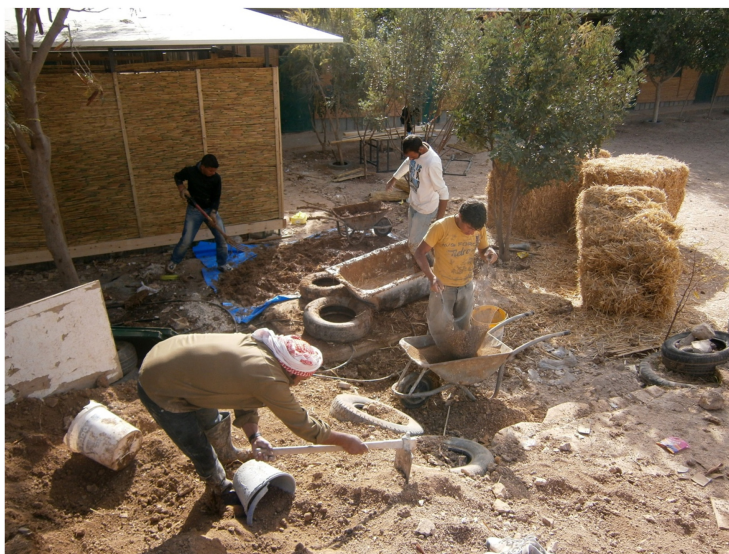
Source(s): Figure reproduced with permission from ©ARCò
