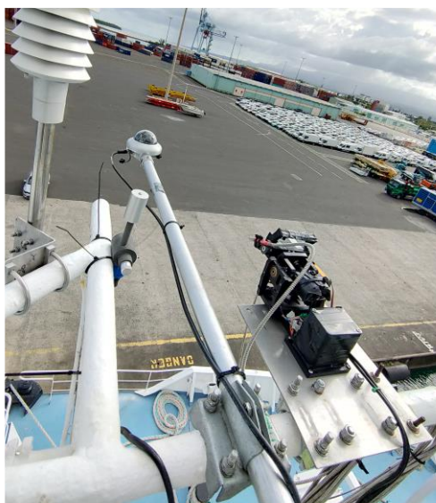
Figure 8. Radiometers (SPN1 and RoX system) installed on the balcony
