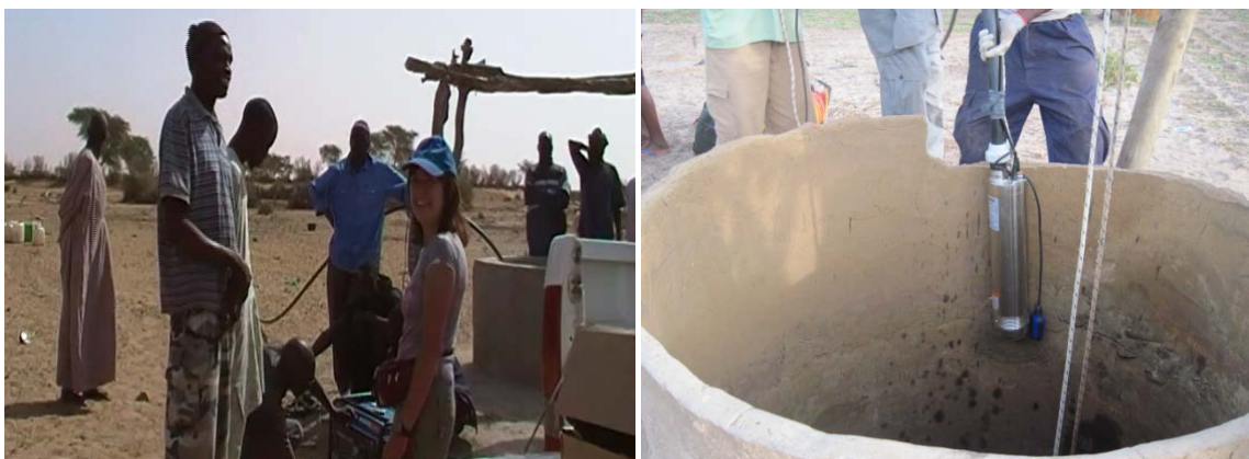
Figure 36 Installation of pump and generator in a large diameter well
