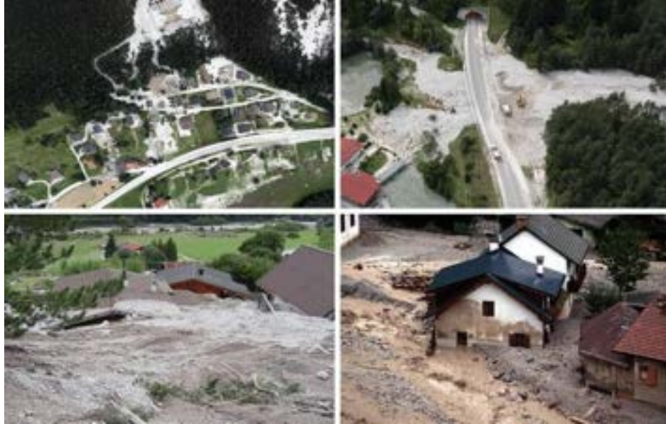
Fig. 1.1: Damage produced by debris flows and flash floods to infrastructure and buildings in the aftermath of the August 2003 event (source: Civil Protection, FVG Region, 2012)
