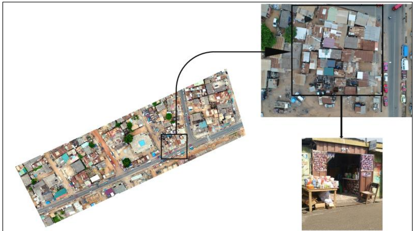
Figure 51: Drone image of container clusters and the risk of fire at New Fadama
