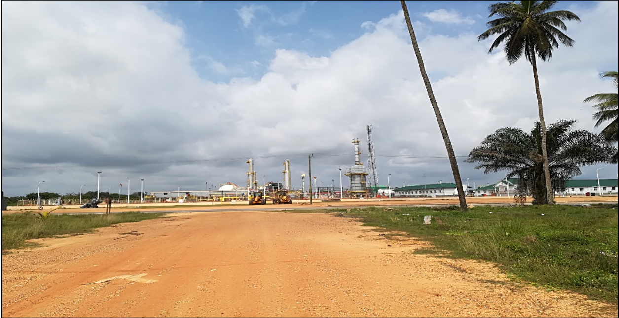
Picture 5.3: Atuabo Gas Plant (Ellembelle District)
