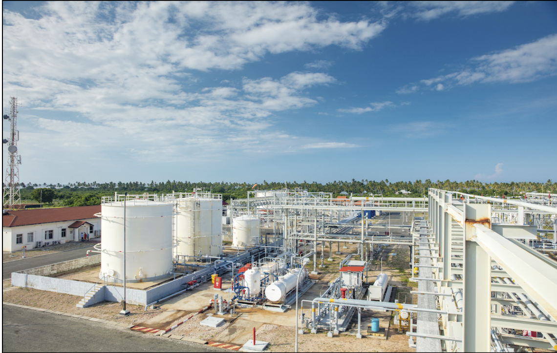
Picture 6.1: Songo Songo Power Plant in Lindi
