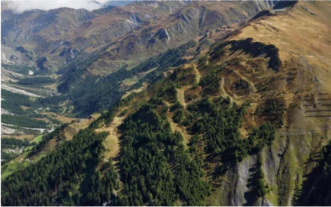
Figure 35 – the upper part of Mont de La Saxe DSGSD, its evident the presents of main scarp, trenches and counter-scarps.
