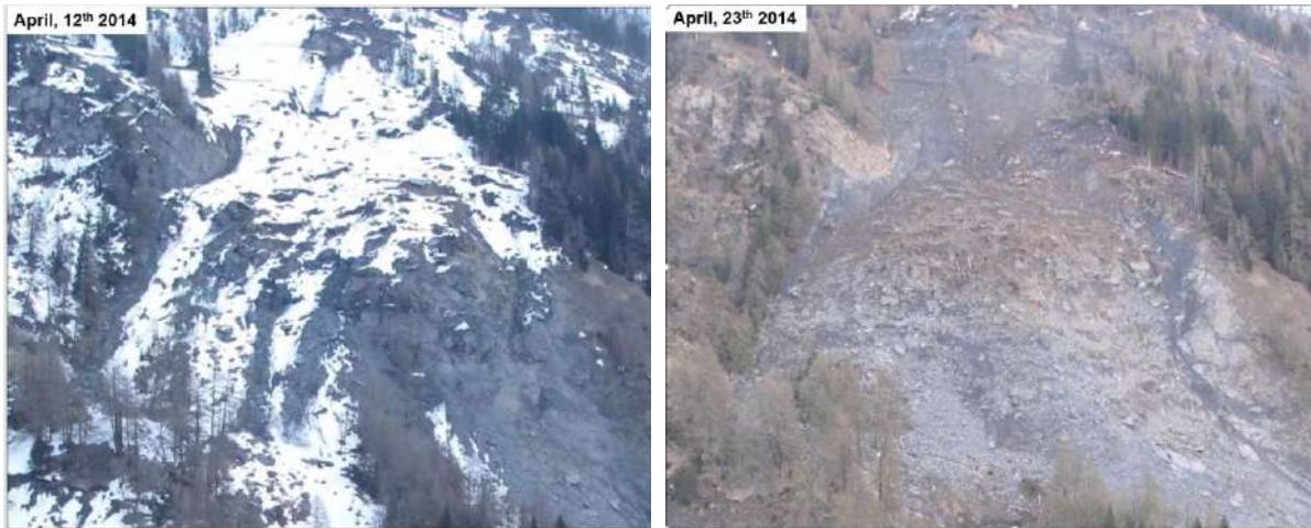
Figure 54 – images from webcam before and after the 2014 collapse, on right-flank of the instability
