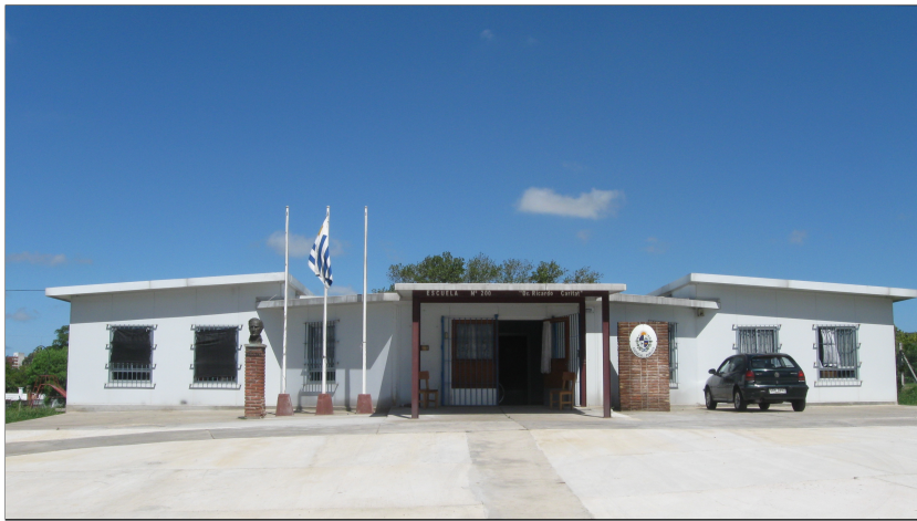
Figure 3.15: The School 200 main entrance
